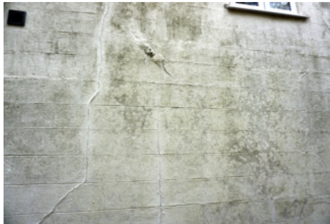
Cracked render and dirty paintwork
