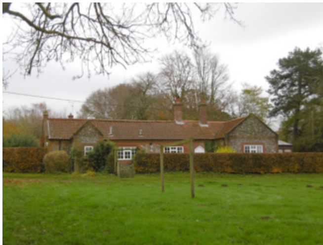
The Old School Room
