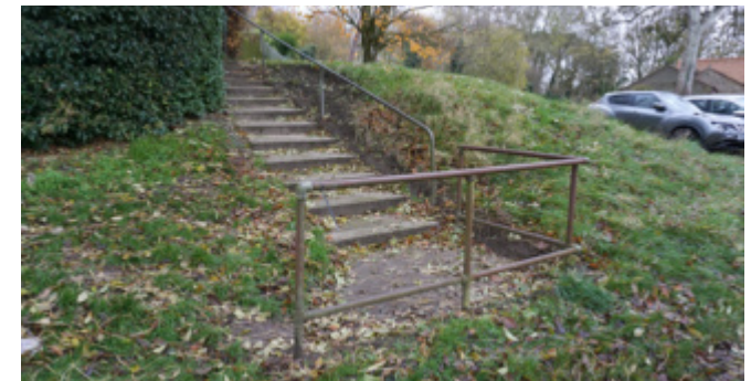
Utilitarian tubular railings
