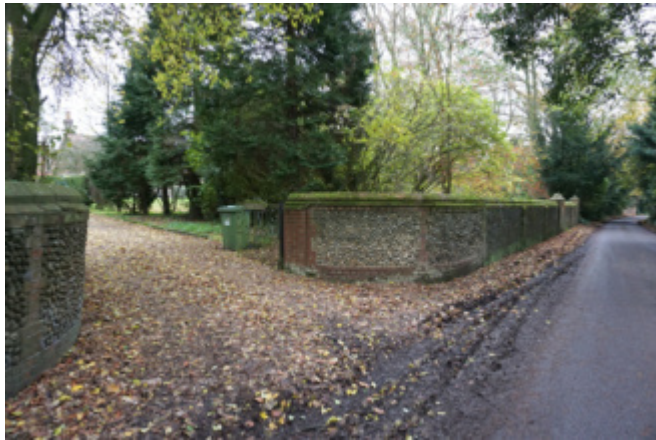
Flint and brick wall with metal gates to Hempstead Lodge
