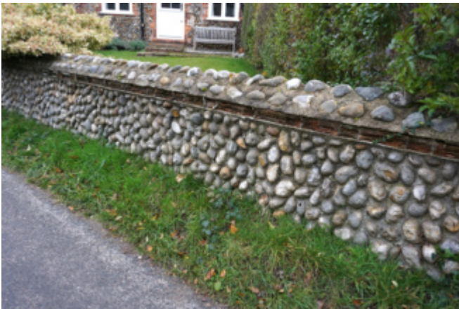
Flint cobble wall
