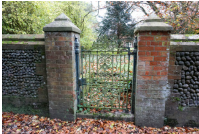
Decorative metal pedestrian gates in a brick and flint wall to Hempstead Lodge
