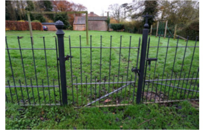
Metal gate and railings to the graveyard
